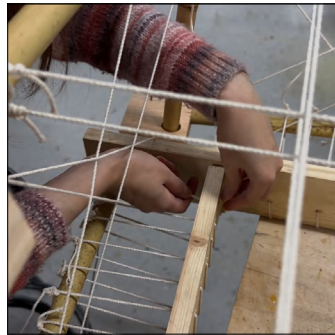
Connect bamboo to the planks with ropes.
