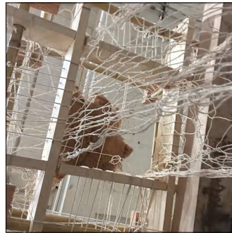
Connect bamboo to the planks with ropes.
