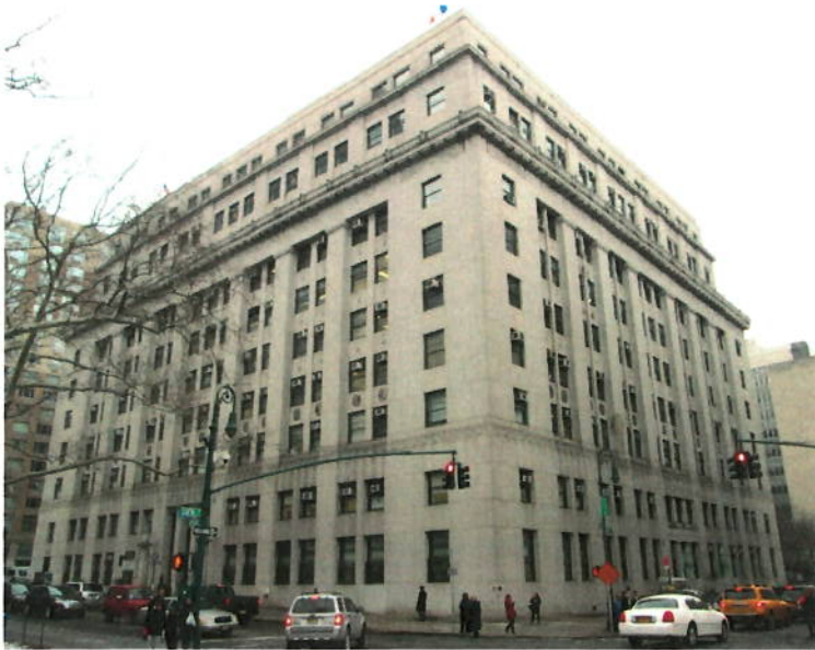
Fig. 2: Health Building, Meyers, 1932-35
