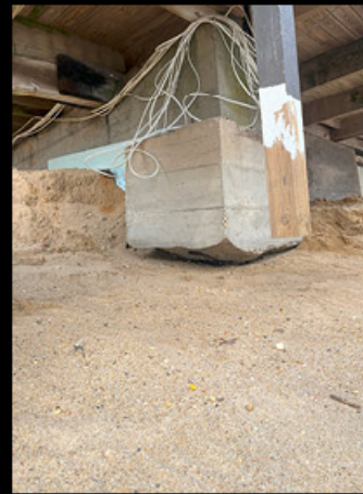
EXPOSED FOUNDATION AT MONTAUK
