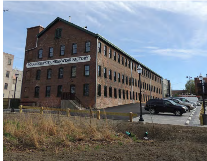
The recently rehabilitated and reopened Underwear Factory, adjacent to the Fall Kill creek and located just off Main Street.
