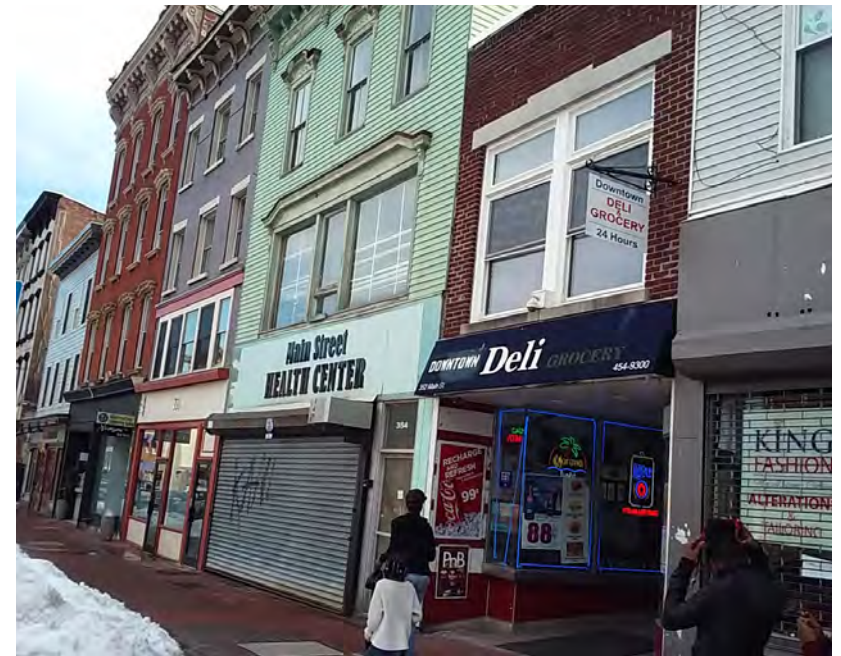
Example of various forms of high and low visual accessibility along Main Street between Academy and Hamilton streets.
