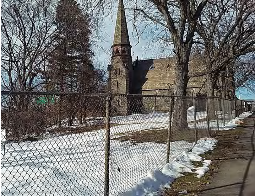
Church of the Holy Comforter, designed by Richard Upjohn in 1860, is an extant, albeit threatened, example of important religious institutions within Poughkeepsie. Route 9 runs adjacent to the church.
