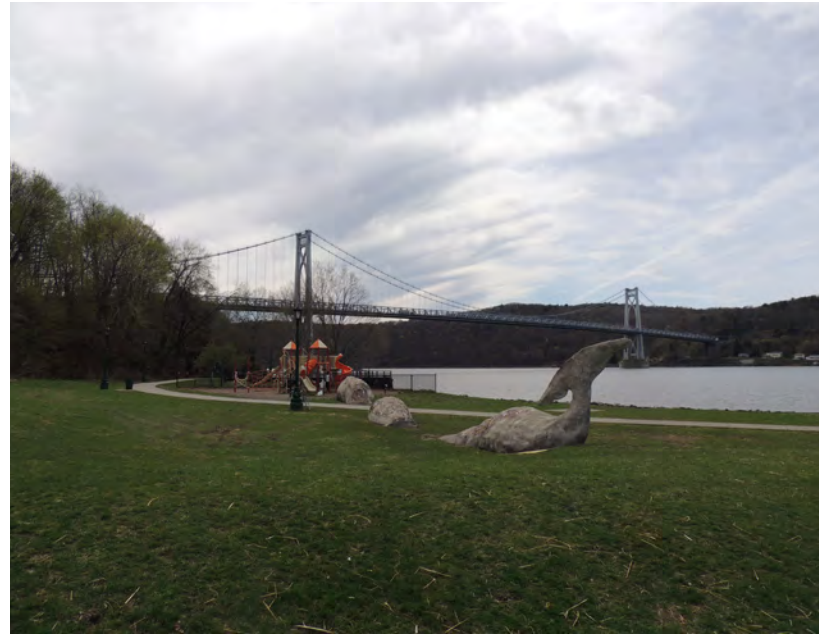
The view of the Mid-Hudson Bridge from Waryas Park.
