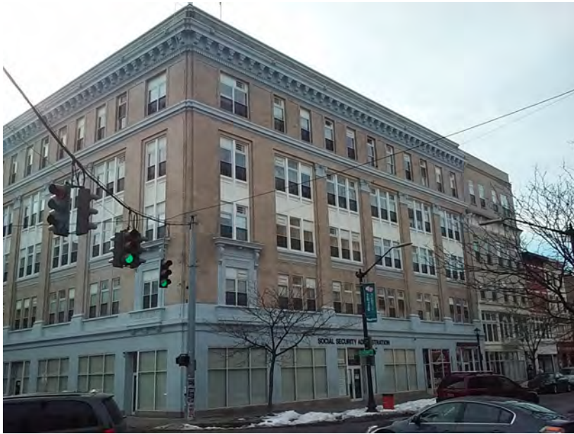
Lucket, Platt & Company Department Store, 332-346 Main Street; Italianate; Year Built: 1923
