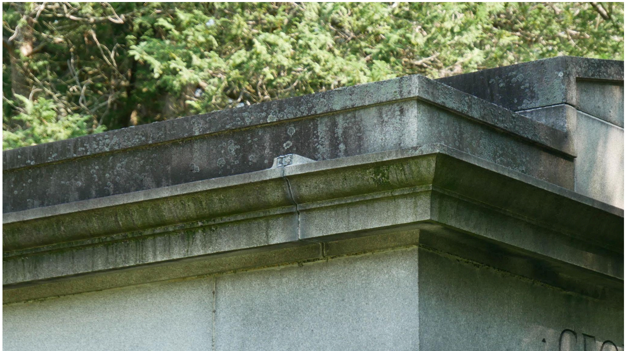
Image 12: Elizabeth Kostina, Lichen and gypsum crust around roof joint , 2024.
