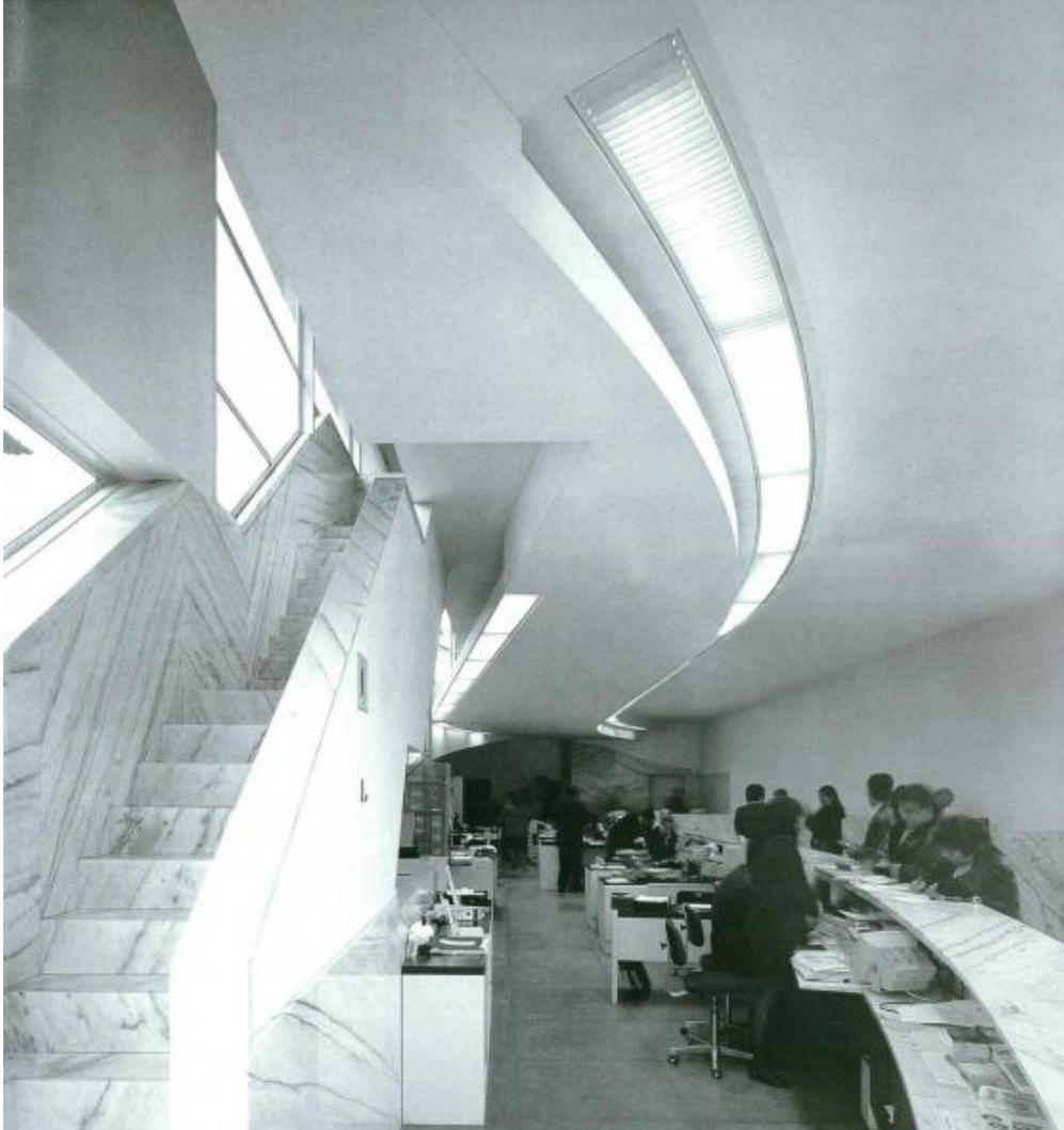
Ceiling lighting (which was combined with the AC diffusers) complement the areas illuminated by natural daylight.
