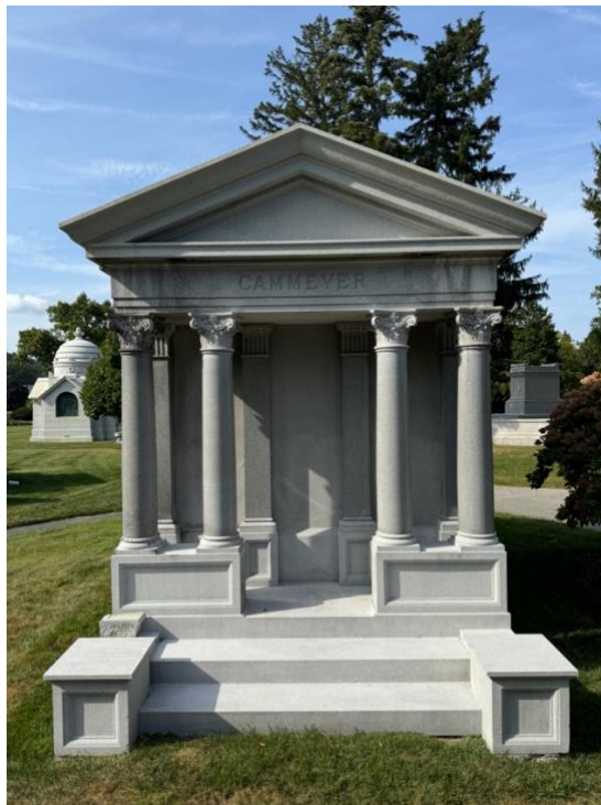
Figure 5: The south elevation of the mausoleum, 2024. Photograph provided by Ashlyn Pause.
