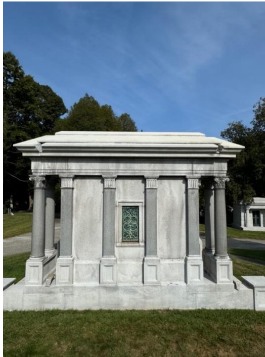
Figure 2: The west elevation of the mausoleum, 2024. Photograph provided by Ashlyn Pause.
