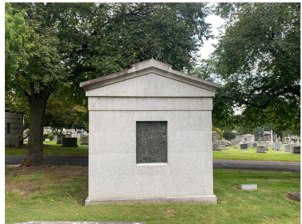
Kane Mausoleum, West Facade, 2021 (Photograph by Kerrian France)
