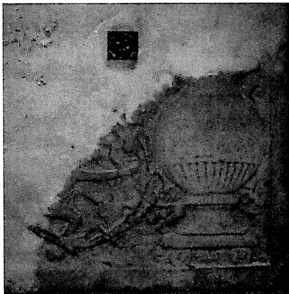
Appendix VIII : Detail of marble crypt covering and stage of deterioration.
