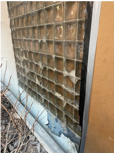
Figure 20 Cracked Glass
