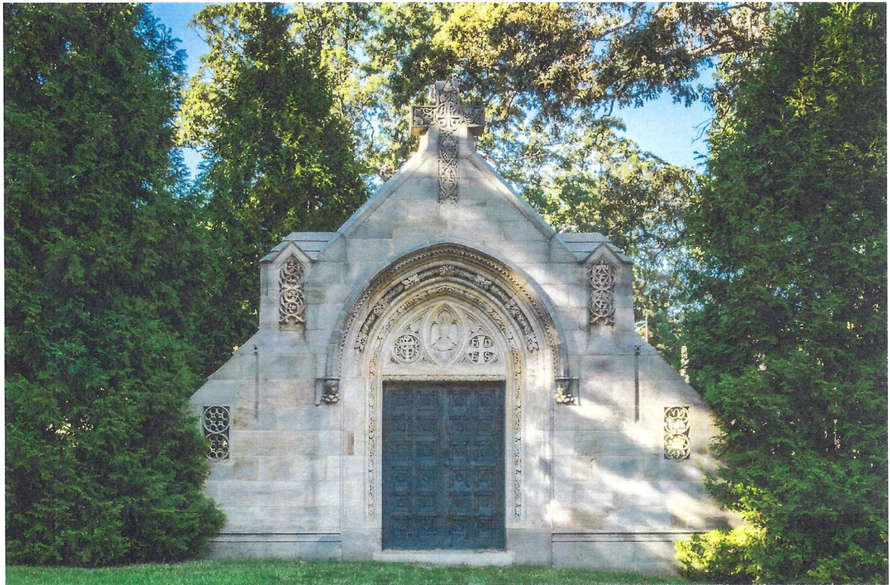
Figure 1 South Elevation taken by Rob Kesack
