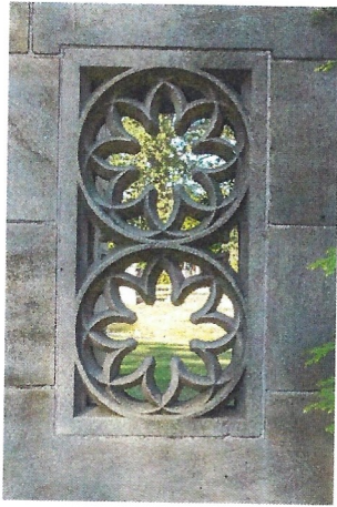
Figure 8 Gothic Tracery in Buttress taken by Rob Kesack
