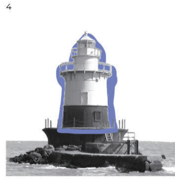
Old Orchard Shoal Constructed: 1893, NY Type: Aquatic Height: 35' (SL: 0') Shape: Conical Foundation: Caisson
