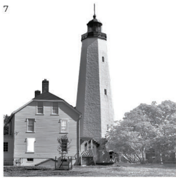
Sandy Hook Lighthouse Constructed: 1764, NJ Type: Terrestrial Height: 85' (SL: 0') Shape: Octagonal Foundation: Masonry
