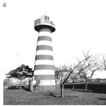
Lefrak Point Lighthouse Constructed: 1872, NJ Type: Terrestrial Height: 50' (SL: 0') Shape: Cylindrical Foundation: Concrete
