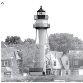
Conover Beacon Lighthouse Constructed: 1856, NJ Type: Terrestrial Height: 45' (SL: 0') Shape: Hexagonal Foundation: Steel Pile
