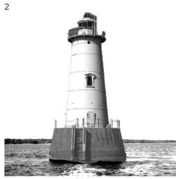
Great Beds Lighthouse Constructed: 1880, NJ Type: Aquatic Height: 62' (SL: 0') Shape: Conical Foundation: Caisson
