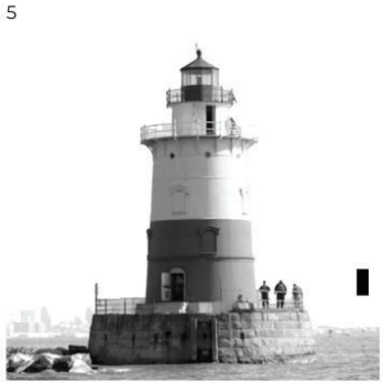
Robins Reef Lighthouse Constructed: 1839, NY Type: Aquatic Height: 45' (SL: 0') Shape: Conical Foundation: Caisson
