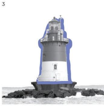
Romer Shoal Lighthouse Constructed: 1838, NY Type: Aquatic Height: 54' (SL: 0') Shape: Conical Foundation: Caisson
