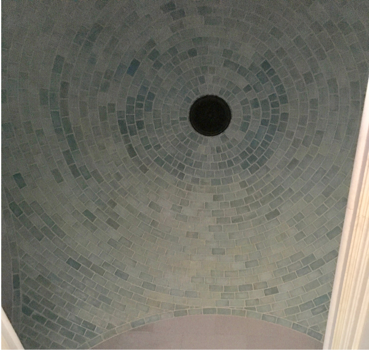
Figure 4: Doherty, Melissa. Light blue Guastavino tile domed-ceiling inside of the Ehret Mausoleum. 2017.
