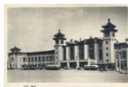
Beijing Railway Station designed by Yang Tingbao with the guidance of Soviet experts in 1959. Occupied "Large roof" style above a modern typology.
