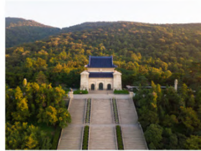
Fig. 3. Sun Yat-sen Mausoleum in Nanjing (1929) designed by Lu Yanzhi.
