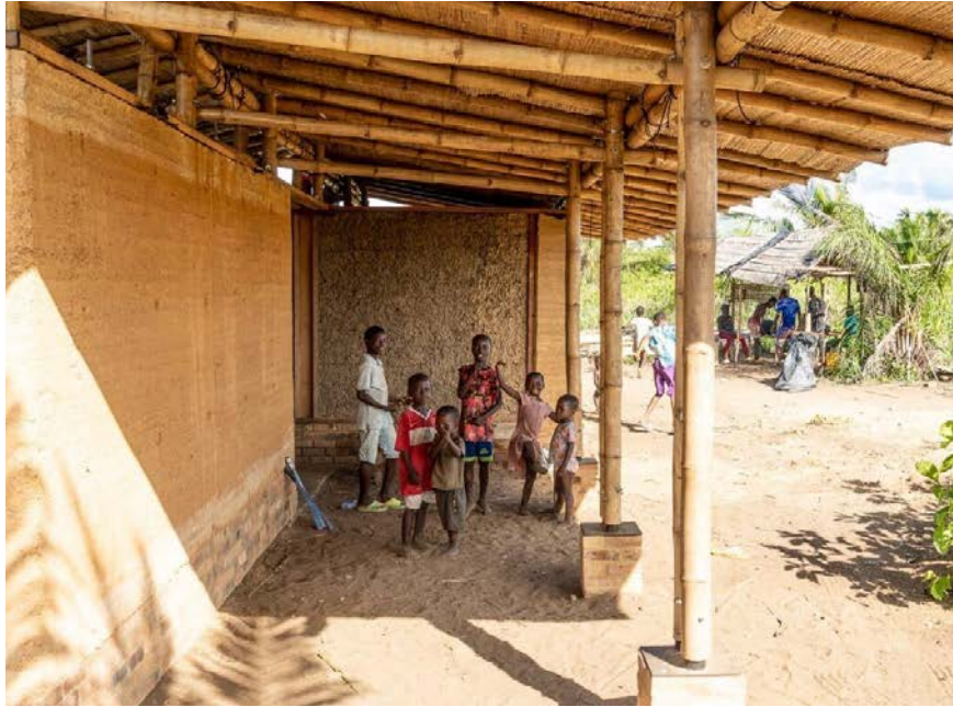
Tadan wall at Zero KM House ISOPTERRA, 2023
