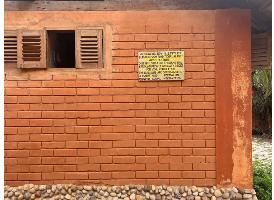
Compressed earth block wall, Kokrobitey Institute Image by Studio Group, October 2024
