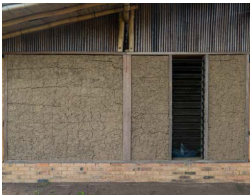
Tadan wall at Zero KM House, Butre ISOPTERRA, 2023
