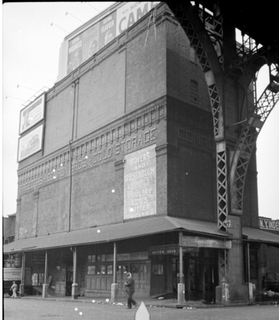
Conron Cold Storage Location at 12th and 131st Street, NYC 23
