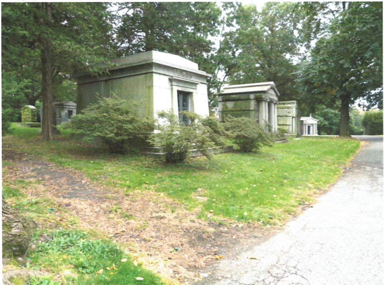
Photograph, Side Façade and Road
