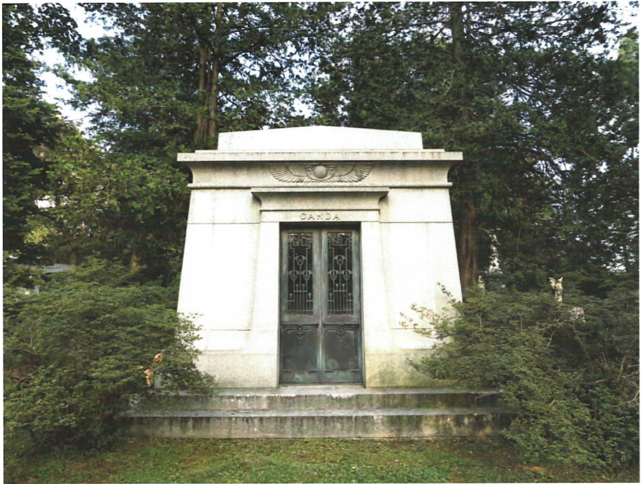
Photograph, Front Façade
